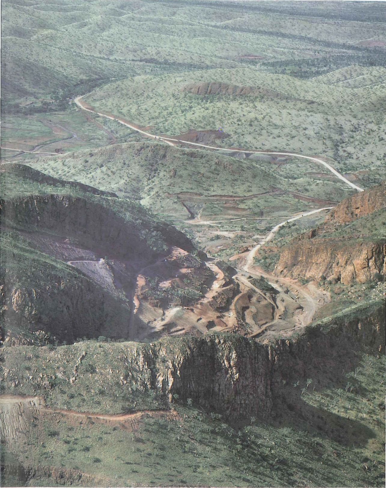
PLATE 12 — The Argyle Diamond Mine in the East Kimberley region. Some 20 million tonnes of overburden must be removed before mining can commence on the diamond-bearing AK-1 kimberlite pipe.
