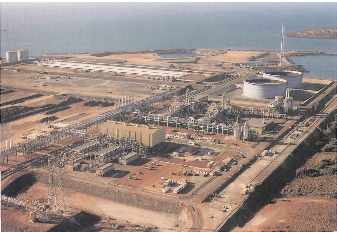
PLATE 11 — The domestic gas treatment plant under construction at Withnell Bay. The plant has a capacity of 10.9 million cubic metres of gas per day for the Western Australian market.
