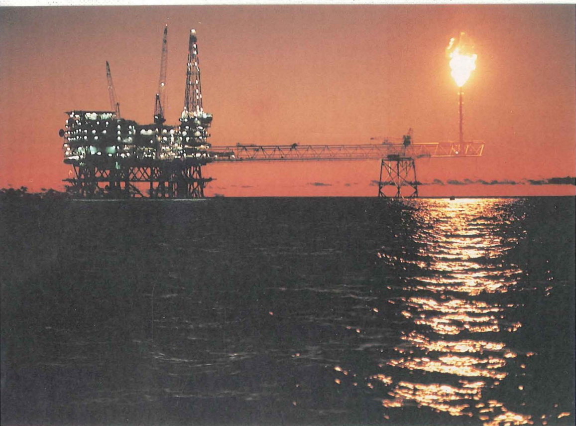
PLATE 10 — The North Rankin 'A' drilling and production platform. A similar platform will be built on Goodwyn field. photograph: Woodside Offshore Petroleum Pty. Ltd.
